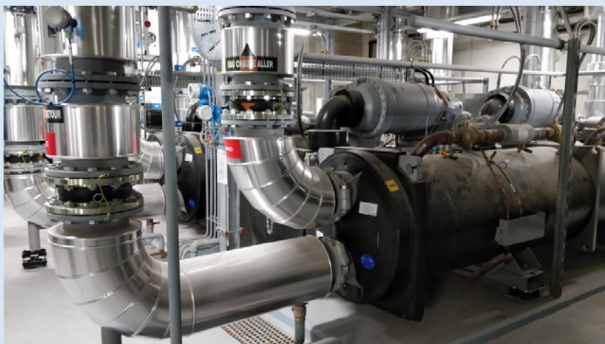
Geothermal heat plant Clichy-Batignolles. Photo: Ute Collier
