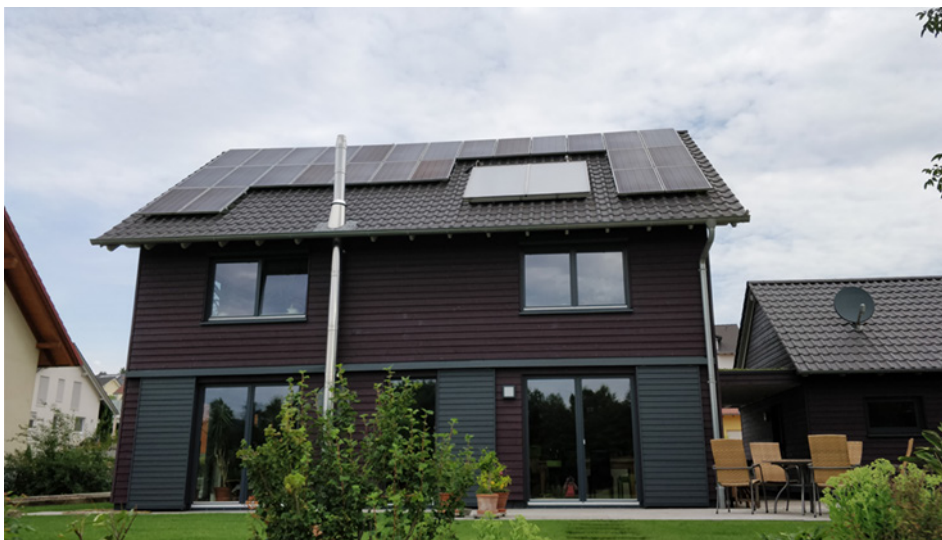
Energy efficient home with solar thermal and biomass heating, Germany
